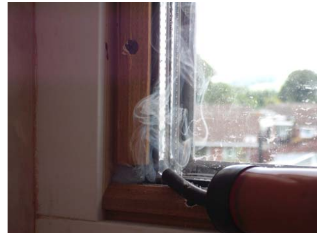
Acceptance test – checking seals around new window in extension
