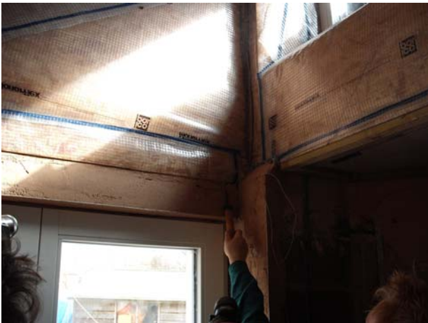
Preliminary test – checking seals between sections of membrane
