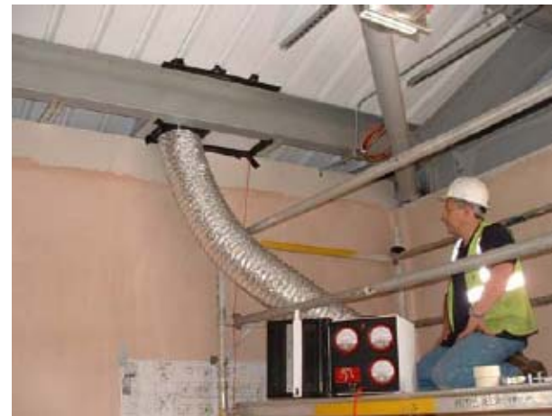
Element testing of the leakage rate along a section of the wall to roof joint
