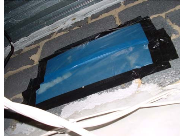
Sample testing of a section of blockwork for leakage
